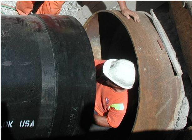
Figure 5 – Preparing Permalok™ Casing for Thread
