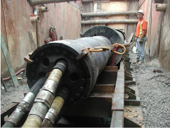
Figure 3. 24" Pipe Hammer Set and Ready
