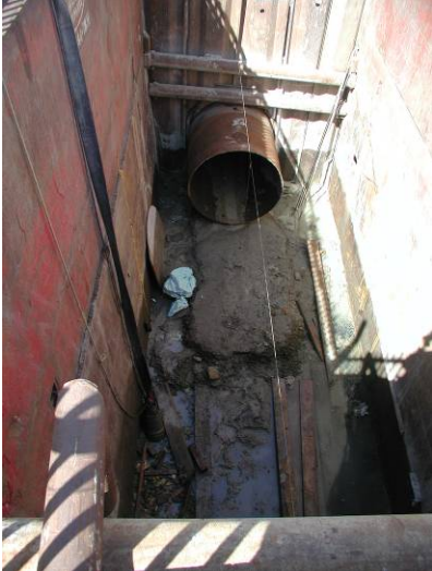
Figure 2 – Hand Mine Set-Up
