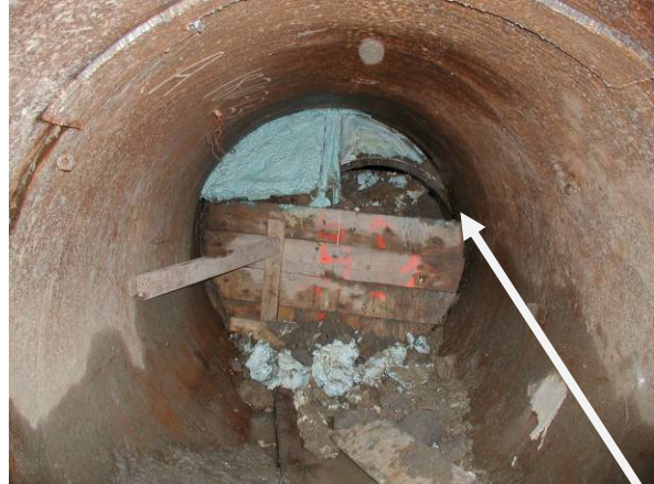
Figure 9 – Ram Connects with Hand Mine Liner
